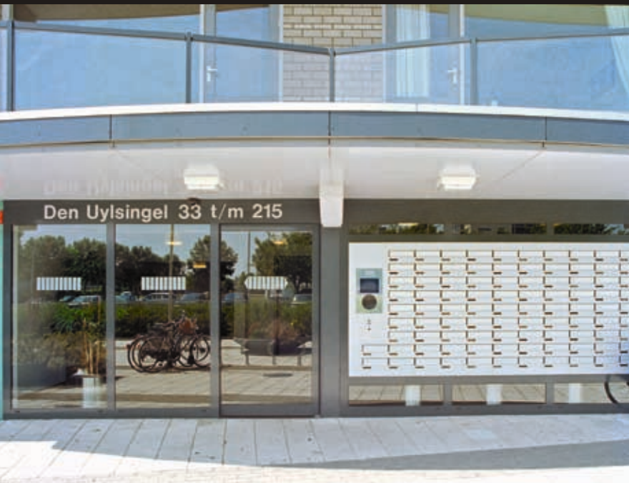
Rotterdam, Dosiatoren, new entrance hall including IRS system
