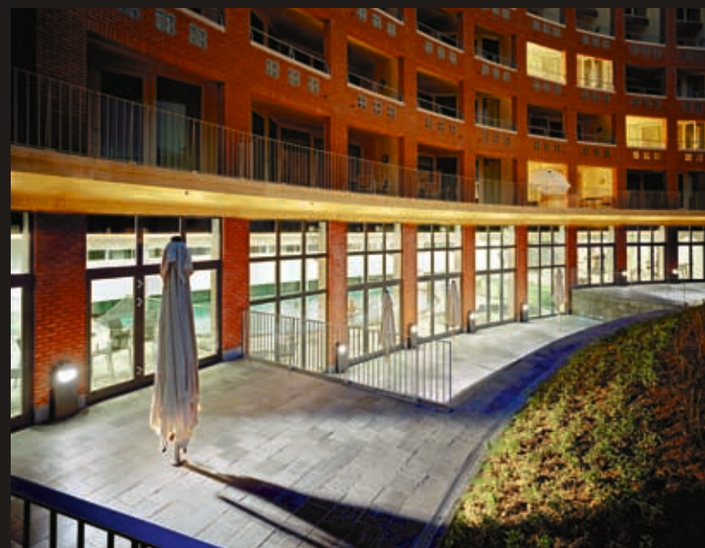
Health Club with swimming pool, fitness centre and sauna in the Cortile project, Céramique Maastricht.
