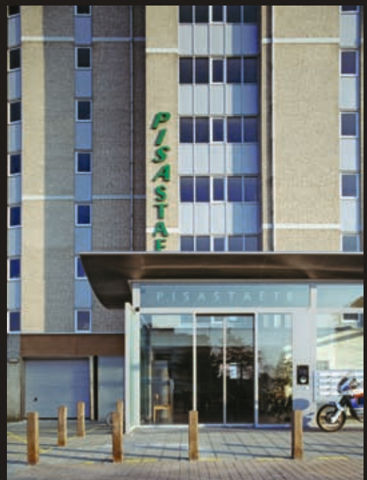
Den Bosch, Pisataete, new entrance hall including IRS system
