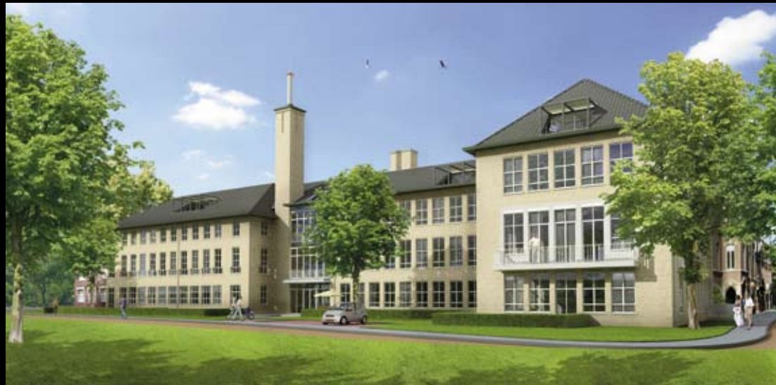
WML building, Maastricht (conversion Hubert Jan Henket en Partners)
